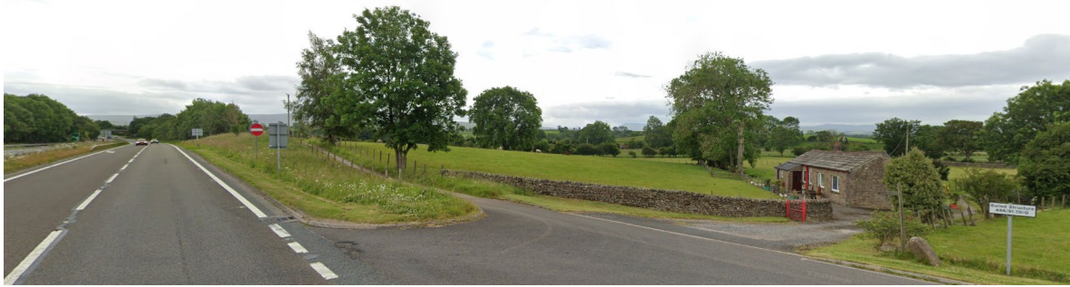
Figure 12 Google Streetview image (photography June 2022) showing access to potential replacement site at Mains House, Brough
